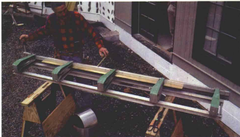
A sheet-metal brake speeds up flashing work. After he checks the measurement at either end of the metal strip, the worker lowers the clamp-bar lever held in his right hand and bends the flashing to the proper angle. An alternative to this portable brake is the site-built one shown below.
